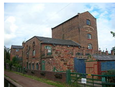
Industrial buildings by the Worcester and Birmingham Canal near Tardebigge , Worcestershire
