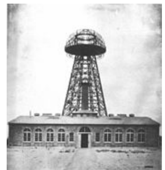
Tesla's Wardenclyffe plant on Long Island in 1904. From this facility, Tesla hoped to demonstrate wireless transmission of electrical energy across the Atlantic.
