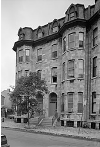
Cope's Pine Street residence
